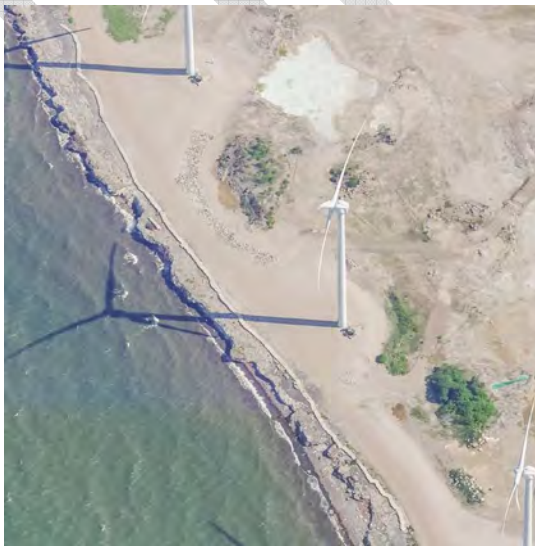
Erosion along the Lake Erie shoreline
