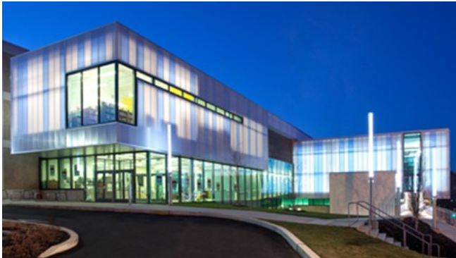
Use of lighting and a clear-glass first floor create a welcoming building day and night, as well as serving as a “billboard” along a major roadway.
