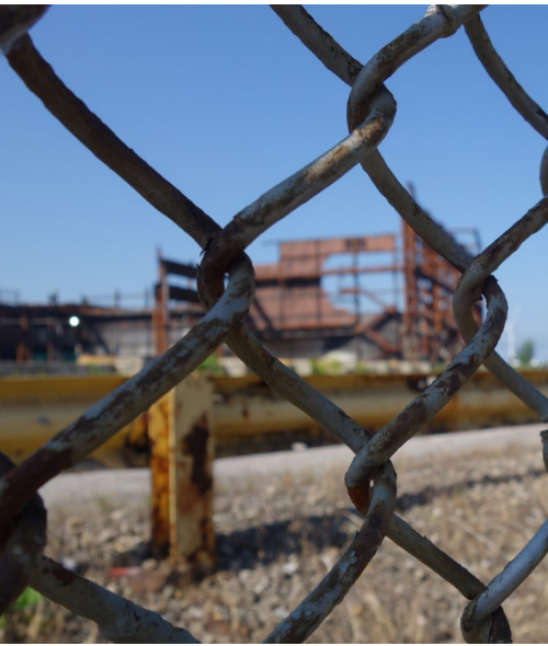
Figure 5.19: Remains following the fire of 2016 on the Hamburg Turnpike
