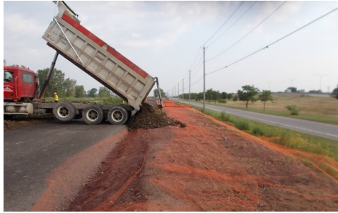
Figure 9.21: Construction on the Shoreline Trail through the Bethlehem Steel Site
