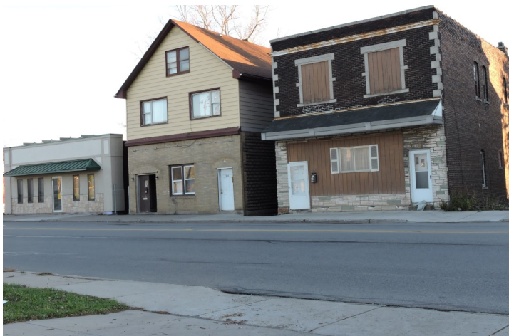
Figure 8.5: Vacant Commercial buildings on Ridge Road
