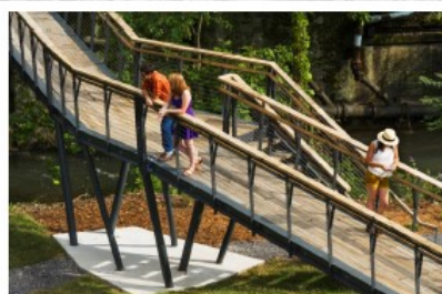
Pedestrian Bridge • Simple bridge structure, crossing railroad tracks • Ramps are provided for bike and wheelchair access
