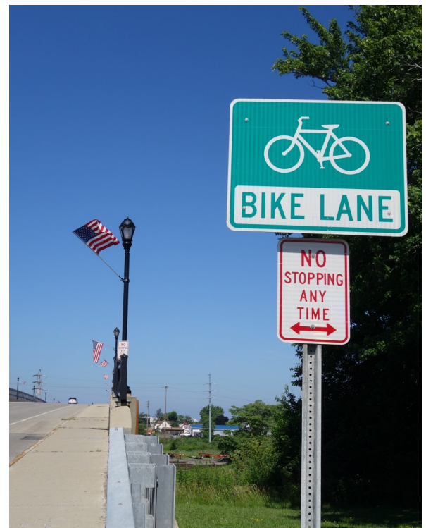
Figure 8.4: Ridge Road Bridge and Bike Lane
