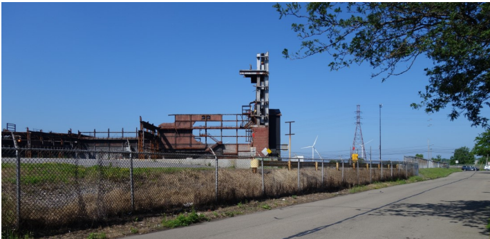
Figure 3.21: What remains after the 2016 fire at Industrial Materials Recycling facility
