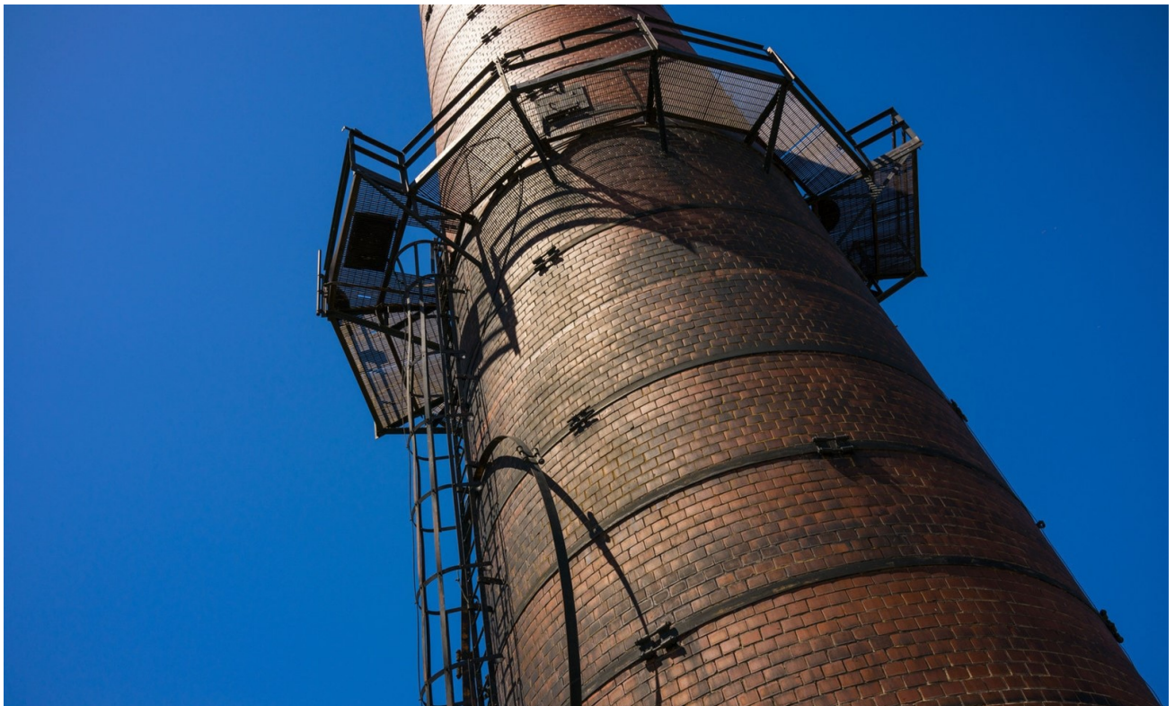
Figure 6.2: Photo: Buffalo News—Vacant Industrial Building within the First Ward BOA
