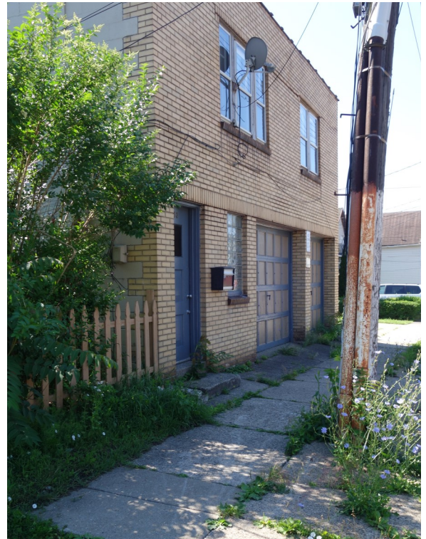
Figure 8.3: Catalyst Site located at Ridge Road and Ingham Avenue
