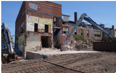
Figure 9.22: Demolition of 100 Dona St. Former Friendship House
